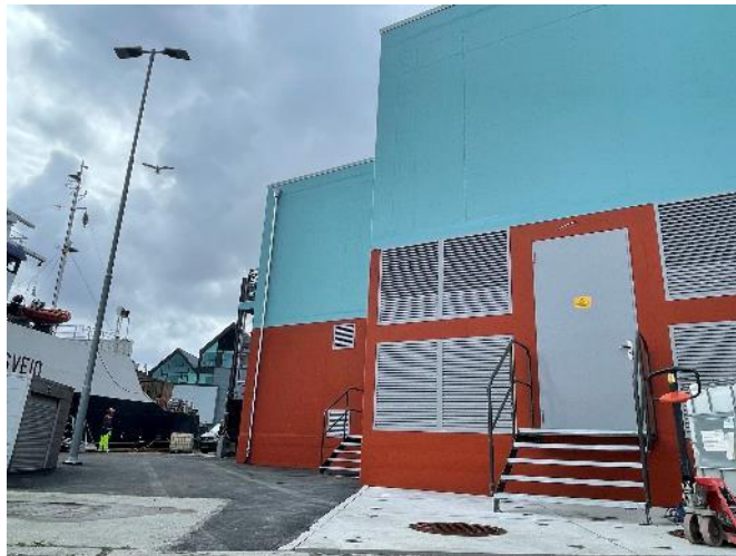
New trafo- and converter building
